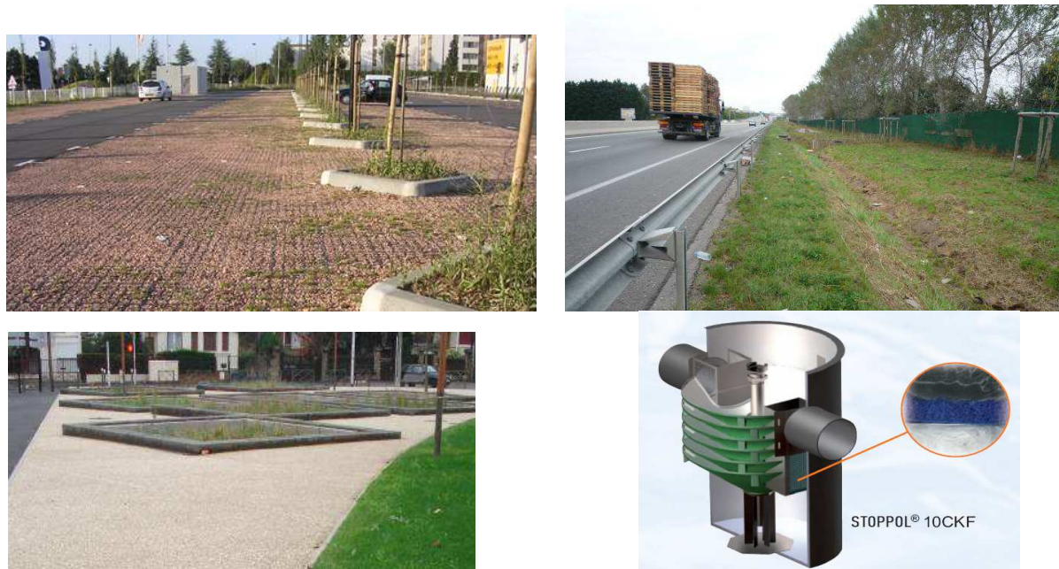
Figure 1 : The four studied pollutant control solutions : (a) pervious parking lot, (b) filter strips and bioretention swale, (c) vegetated sand filters, (d) compact sedimentation/filtration/adsorption device
