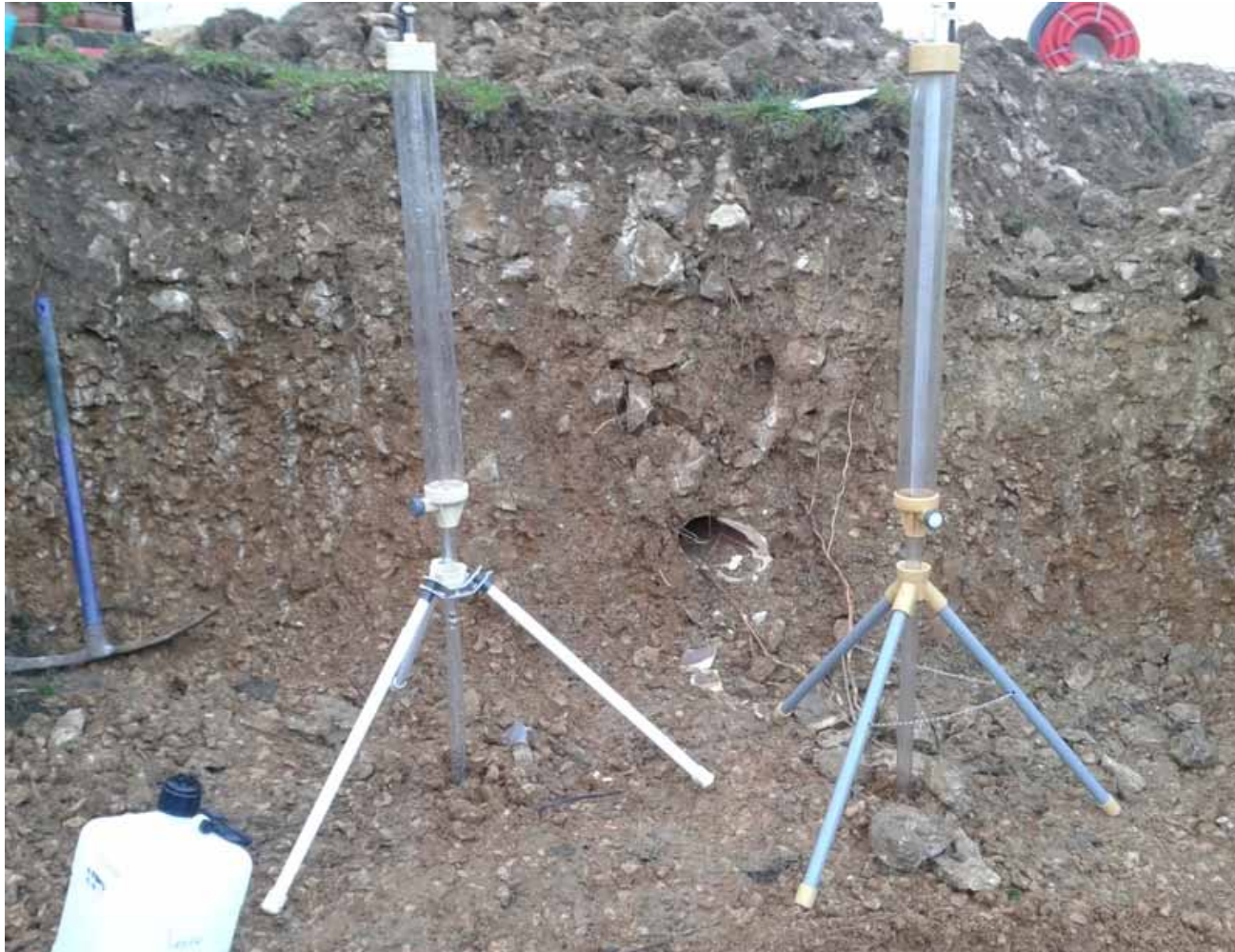
Hydraulic conductivity tests by Guelph permeameter at the bottom of the excavation
