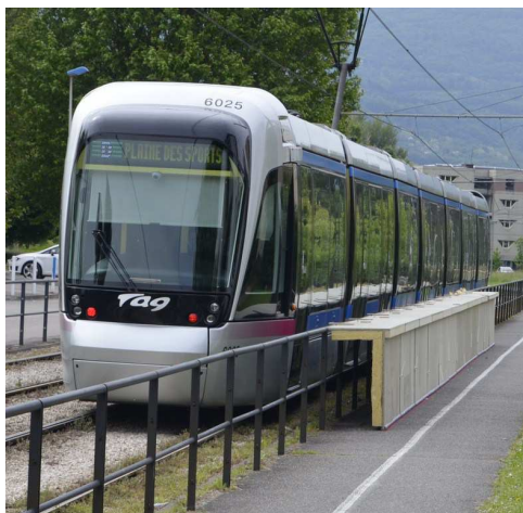
Figure 8.3: View of the noise barrier prototype with a Alstom Citadis 402 tramway of the Grenoble B line passing-by. The length of the barrier is about 22 m, whereas the tram is about 43 m long.
